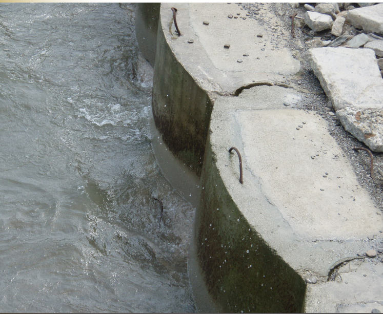
Concrete block seawall along Ohio's shore.
